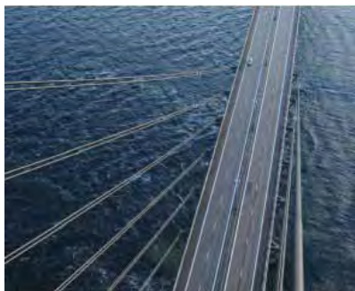
Fig. 1 The cables of the Öresund bridge (Sweden) underwent large rain-ice-wind induced vibrations (galloping).
